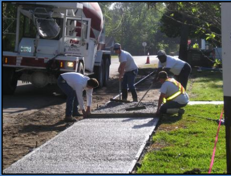
Crews installing new sidewalks in Alachua.
