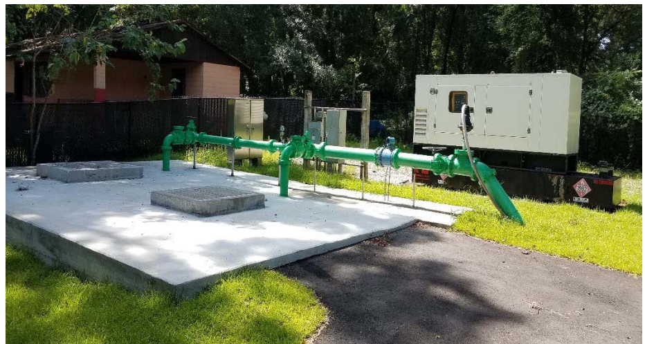
Lift Station #1, the City's Primary Lift Station, was originally installed in 1976.
